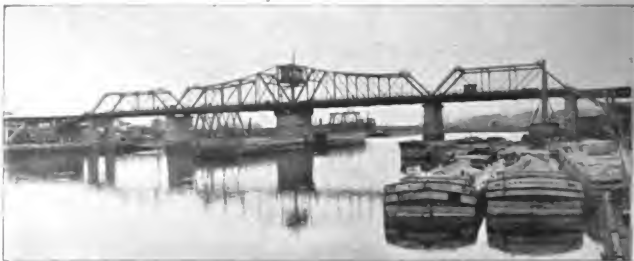
HARLEM RIVER AND SECOND AVENUE BRIDGE, AT 129TH STREET.
